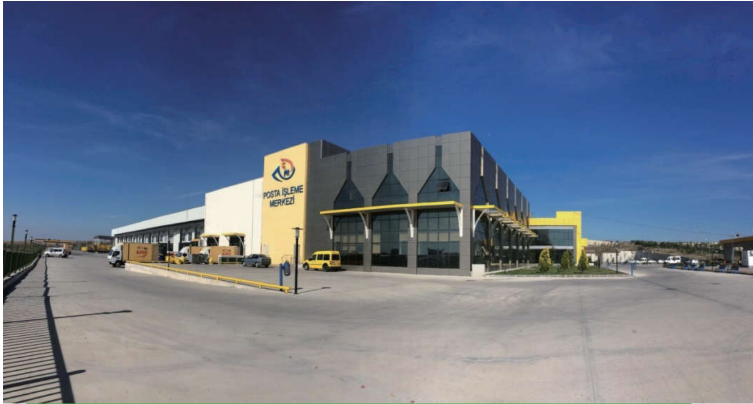
PTT Istanbul office and operation center in Turkey, total VRF capacity 2500kw
